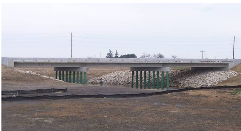
Figure 2. Completed replacement bridge on 120 th Street.
