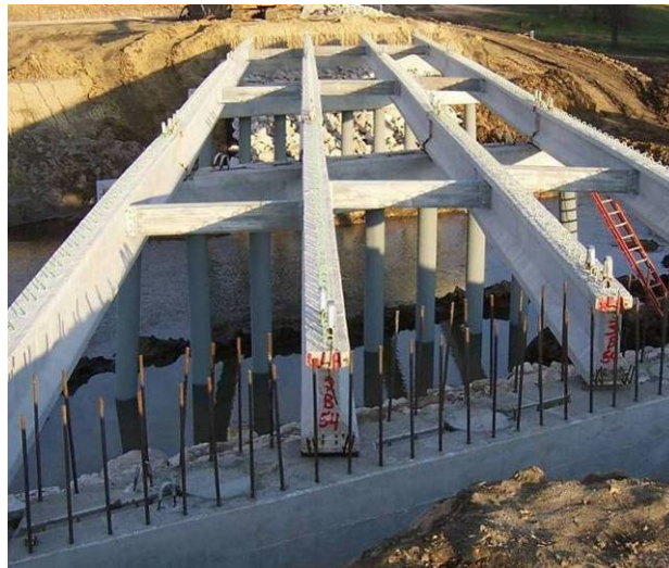
Figure 128. Erected bridge girders, October 24.
