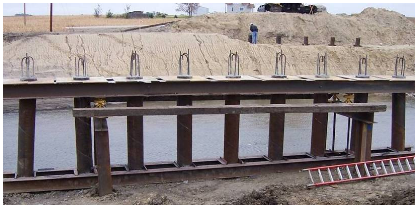
Figure 115. Pipe pile reinforcement for pier cap connection, October 4.
