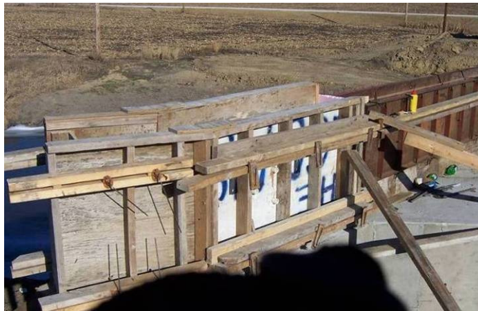
Figure 145. Barrier rail formwork, December 8.
