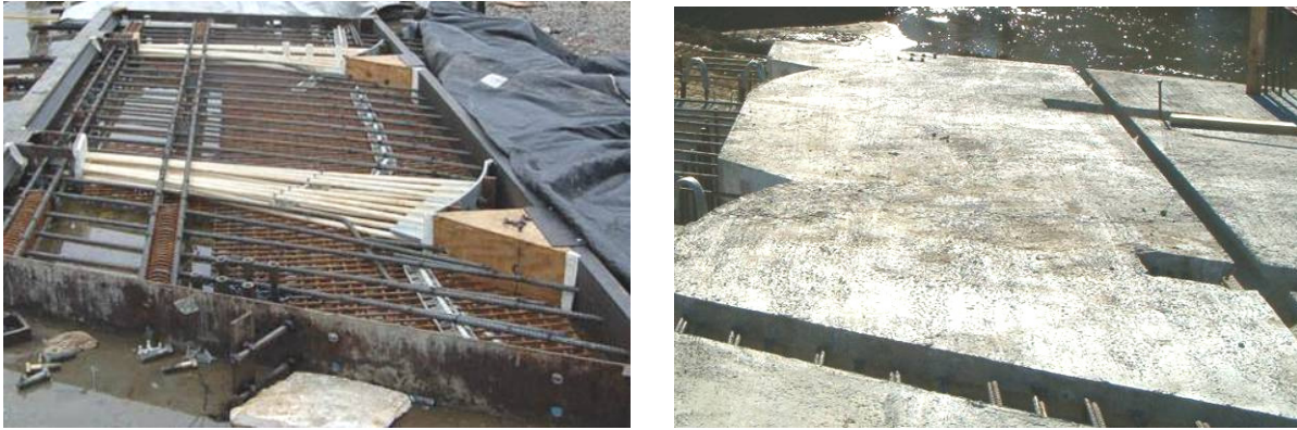
a) end panel reinforcement
