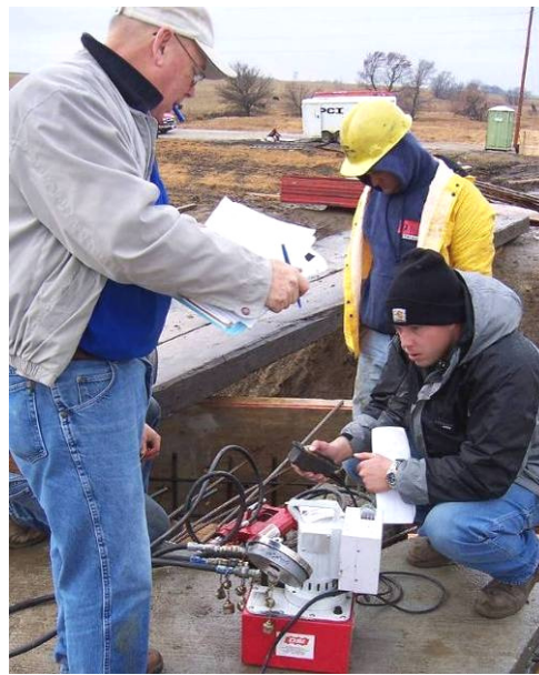
Figure 140. Post-tensioning in progress, November 28.
