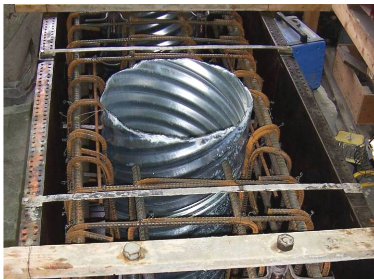
Figure 27. Pier cap reinforcement.
