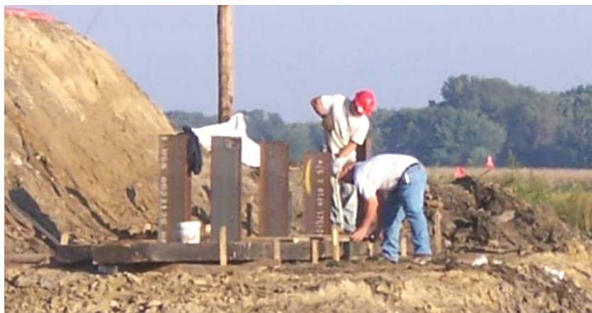
Figure 109. West abutment piles, driven and channels being blocked, September 15.
