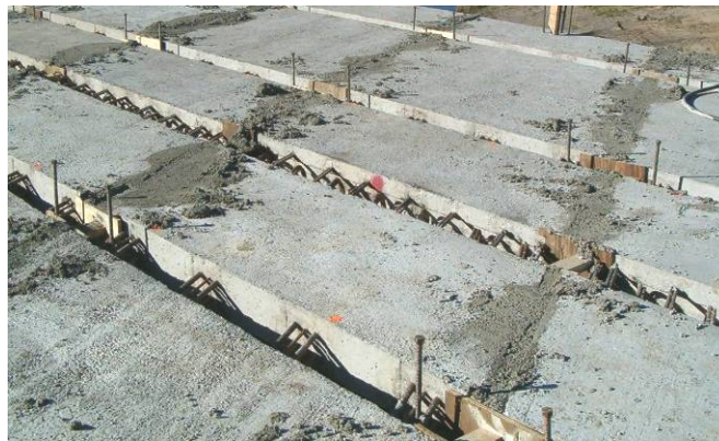
Figure 135. Several transverse joints before finishing, November 8.
