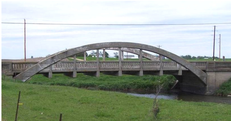
Figure 102. Previous bridge on 120 th Street, July 19.
