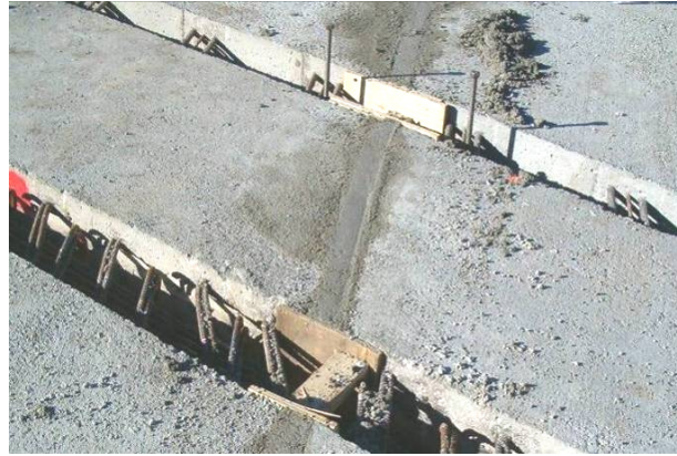
Figure 136. Finished transverse joint, November 8.
