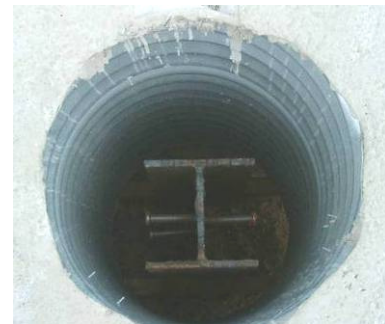
b) H-pile in the abutment
