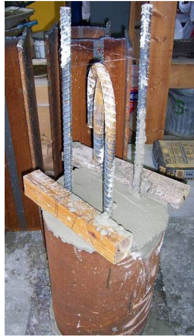
b) pipe pile after placing concrete
