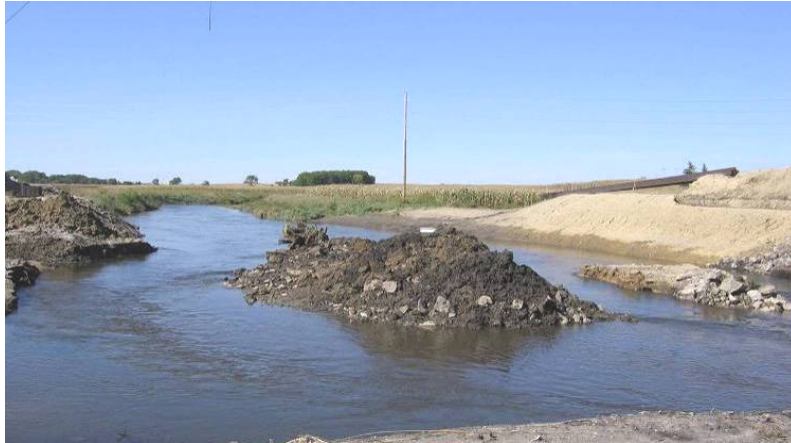
Figure 110. Bridge site on September 20.
