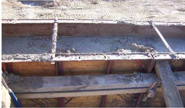
Figure 147. Barrier rail before final finishing, December 8.
