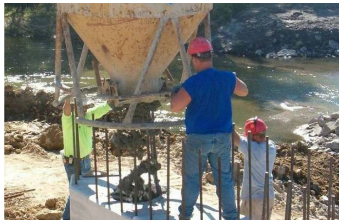
Figure 121. Concrete being placed in the east abutment, October 5.
