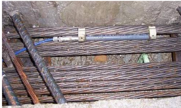
Figure 84. PT strand vibrating wire gage.
