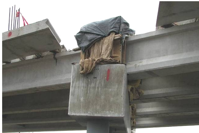
Figure 132. West pier diaphragm covered with burlap and plastic, November 4.
