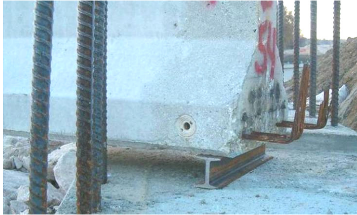
Figure 127. Steel beams used to support the girders, October 24.
