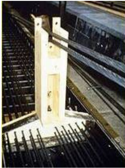
Figure 3. Bulkhead in a prestressed concrete casting bed.
