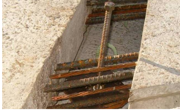
Figure 130. Deck panel leveling screw, October 26.
