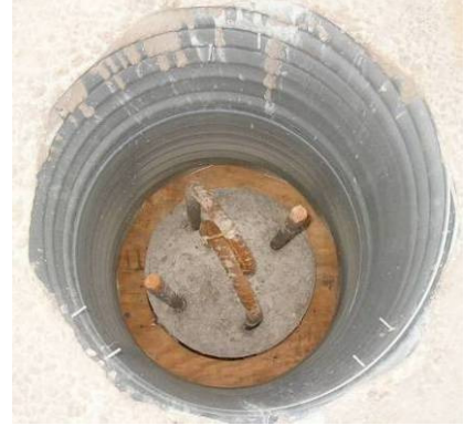
b) pipe pile in the pier cap
