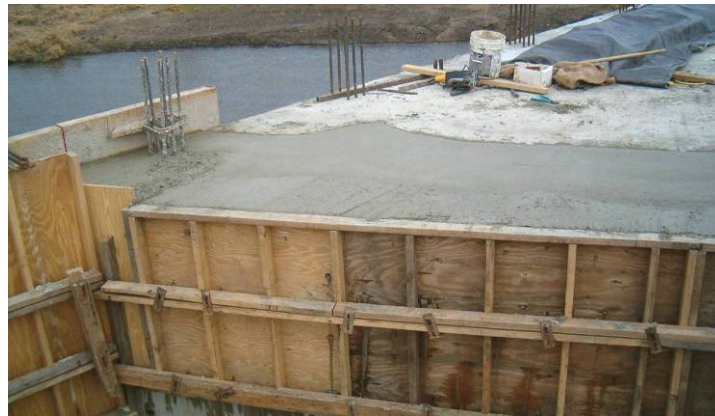
Figure 144. West abutment and wingwall, placed and finished, November 29.
