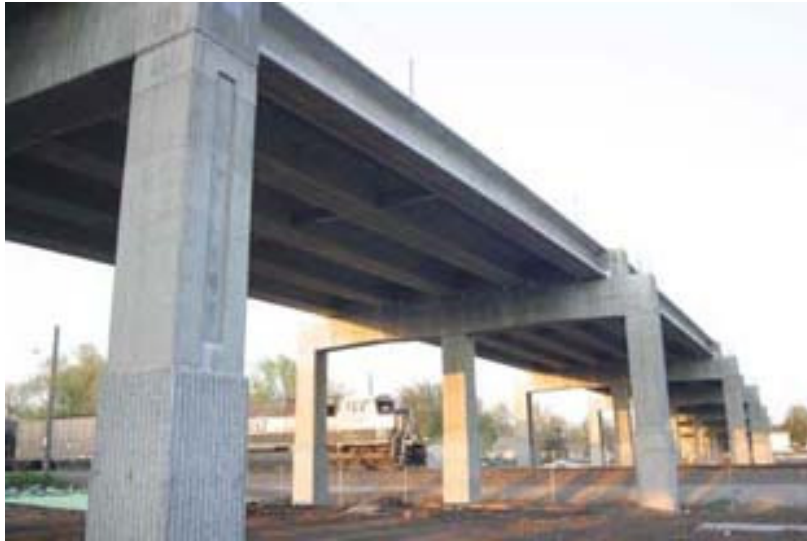
Figure 8. Bridge pier cap located Lincoln, Nebraska.
