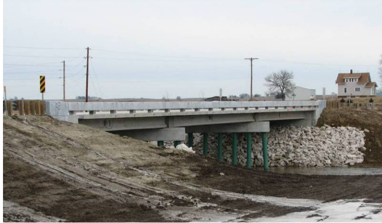
Figure 151. Completed bridge, December 27.
