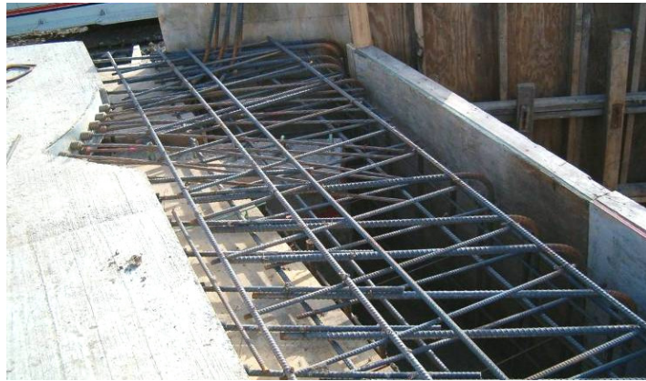
Figure 143. Reinforcement in the west abutment cap, November 29.
