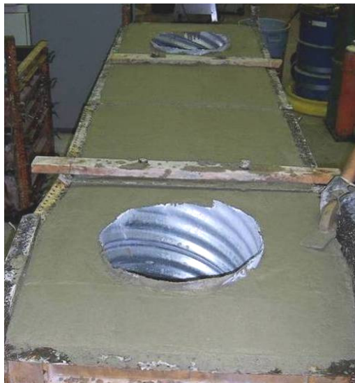
Figure 33. Abutment 6 after hand-finishing.
