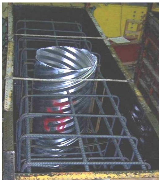
Figure 17. Completed formwork with the CMP for the first abutment test specimen.
