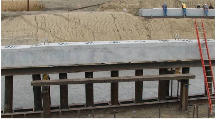
a) pier cap in place
