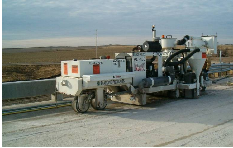
Figure 148. Bridge deck grinding equipment on site, December 27.
