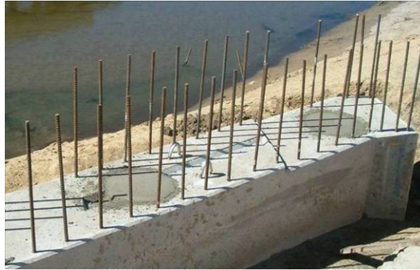
Figure 122. Finished specialty concrete in the east abutment, October 5.
