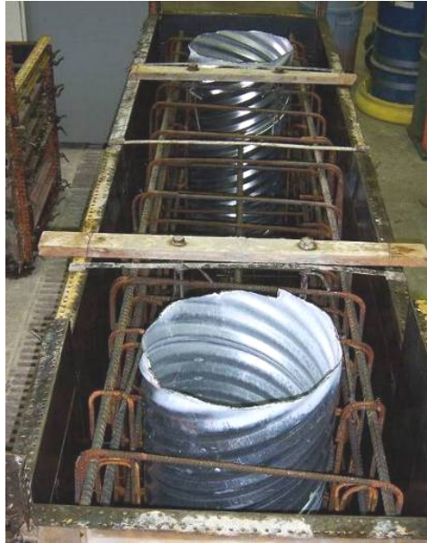
Figure 32. Finished reinforcement and formwork for ADC1.
