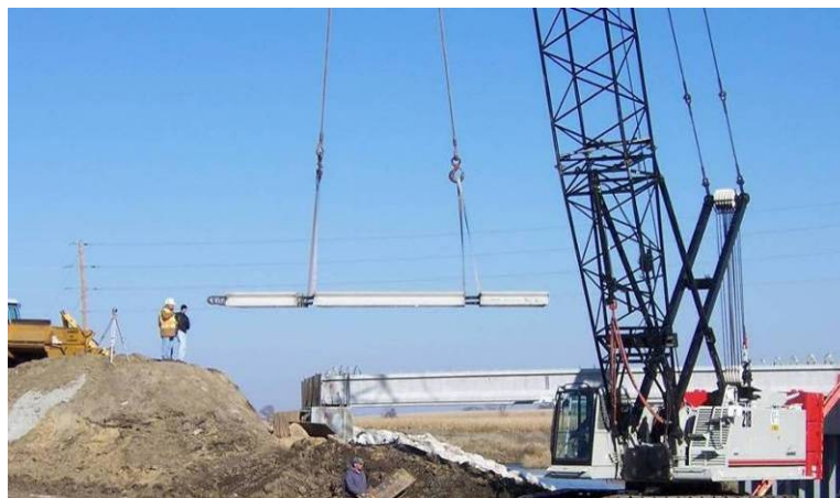
Figure 129. Deck panel being reset on the bridge girders, October 25.
