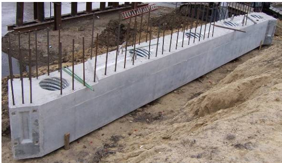
a) abutment in final position
