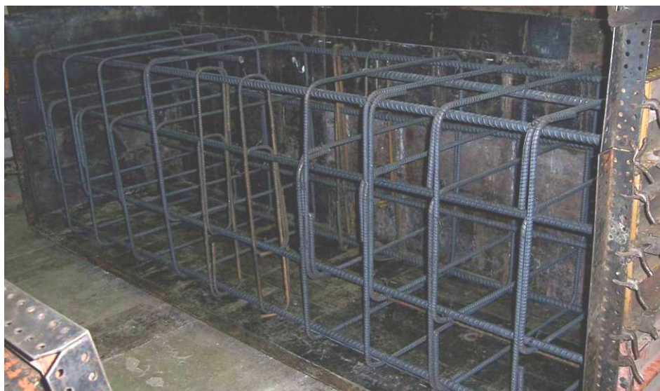
Figure 16. Single pile abutment specimen reinforcement placed in the formwork.
