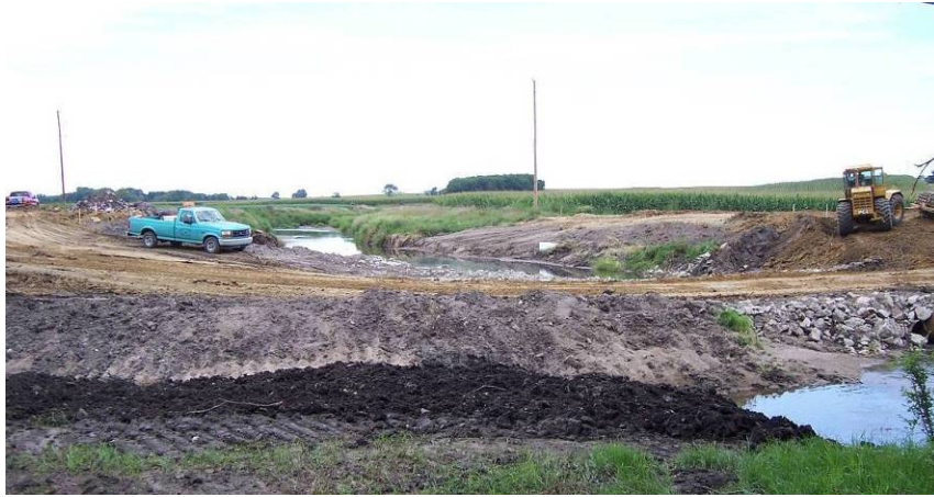
Figure 105. Cleared bridge site, August 7.
