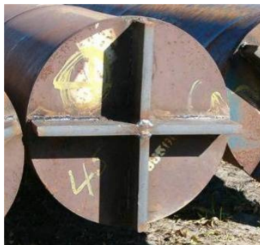
Figure 113. Steel pipe pile driving point, September 28.
