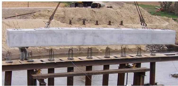
Figure 118. West pier cap being lowered into place, October 4.
