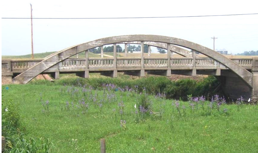
Figure 1. Marsh Arch bridge previously on 120 th Street.
