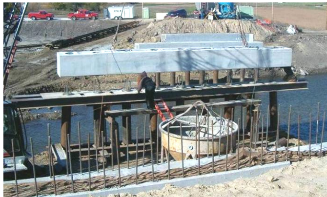
Figure 125. East pier cap being set, October 12.
