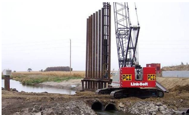
Figure 123. East pier pipe piles being driven, October 10.
