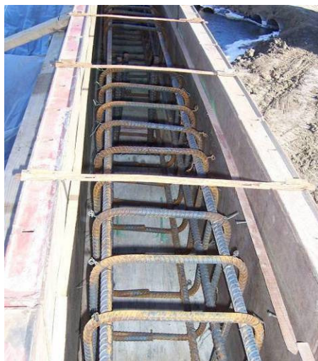
Figure 146. Barrier rail reinforcement, December 8.
