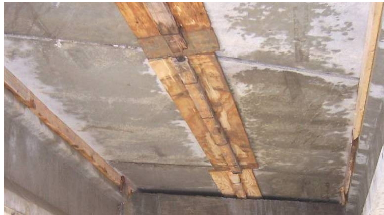
Figure 141. Longitudinal joint formwork, November 28.
