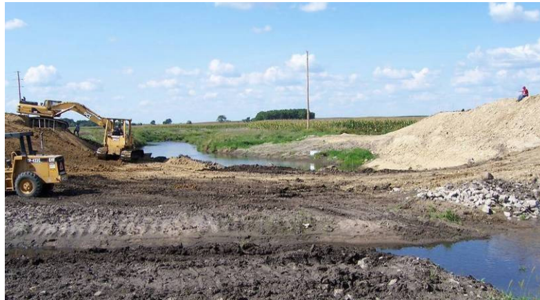
Figure 107. West bridge abutment site prepped for pile driving, September 5.
