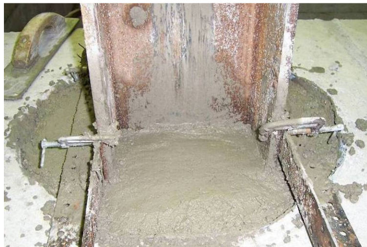
Figure 23. H-pile after being grouted in place.
