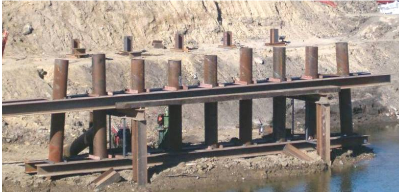
Figure 114. West pier and west abutment piling, September 28.
